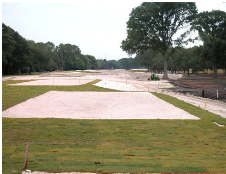
Figure 1: Capping tees and fairways with sand can greatly improve the growing environment for turf, especially on sites with poor-quality soils or irrigation water.
