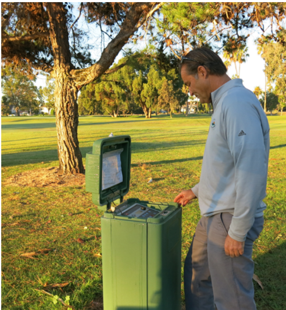
Checking the satellite controllers and central computer for backup programs and accurate run times should be done at least once every month.
