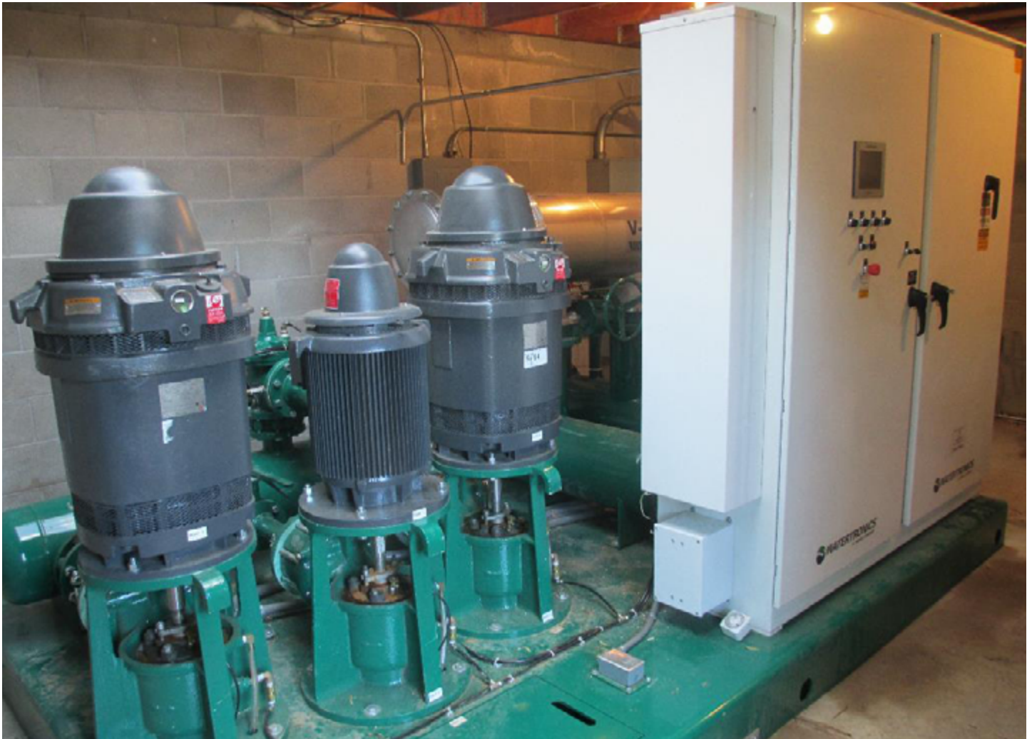
Pumps are the heart of an irrigation system. Semiannual maintenance of electrical and mechanical components by a trained technician ensures efficient operation.
