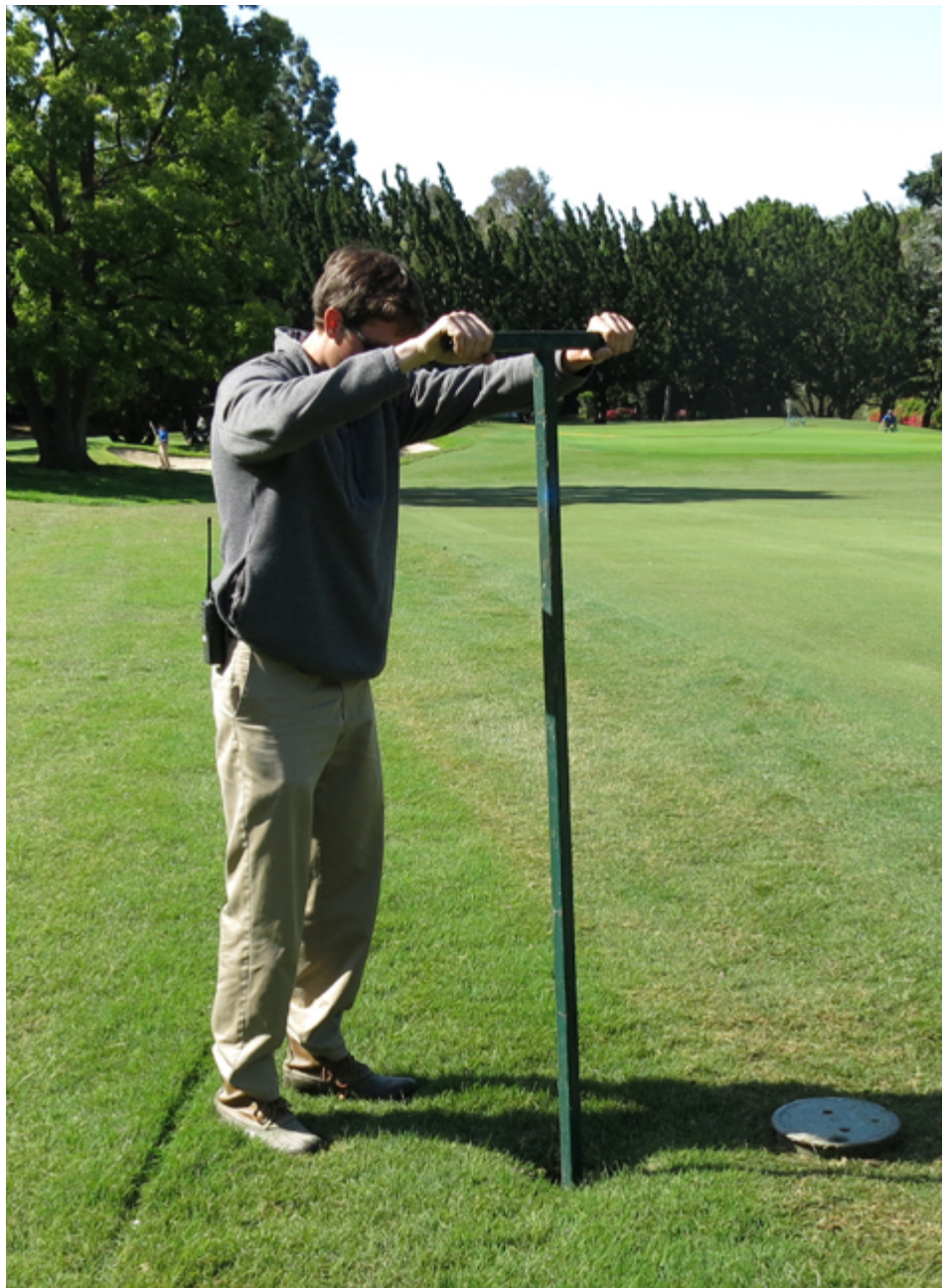
Isolation valves and drain valves should be exercised annually to prevent them from sticking open or closed.
