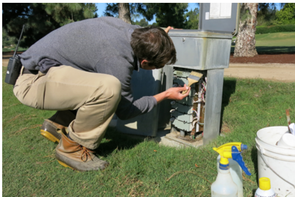
Clean field satellite controllers quarterly by dusting, removing cobwebs, and replacing insect repellent. This can greatly extend the life span of electrical components.
