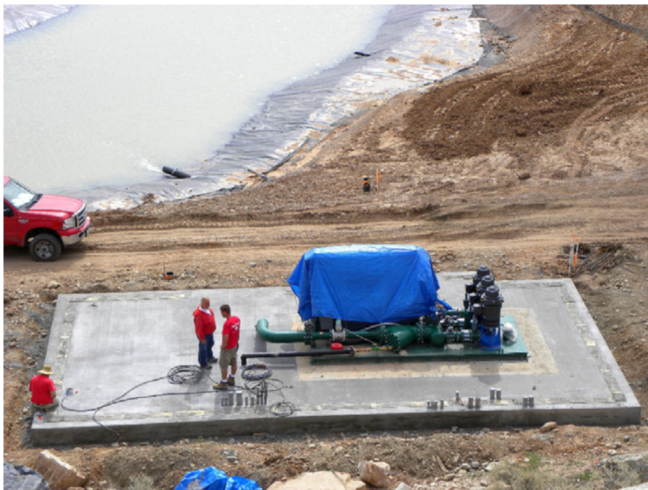
The new Rainbird pump station and pad for the new building in March of 2010.
