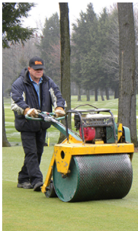
New washed sod is being rolled carefully not long after installation to begin to stabilize and smooth the surface.
