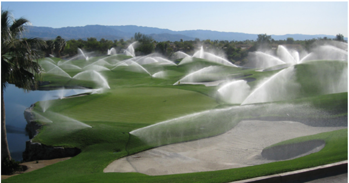
Irrigation technology today allows for very precise application rates and accuracy when irrigating fairway and rough areas.
