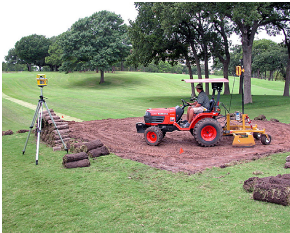
Projects like tee box rebuilding and even re-leveling a tee surface require not only a well-researched plan and experienced crew, but they often may take specialized equipment, like this laser level and box-blade.
