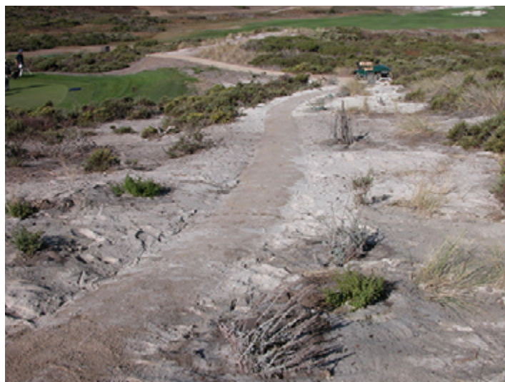
Paths composed of stabilized sand or soil can be incorporated into turf reduction areas to help facilitate movement of golfers, carts, and equipment through the golf course.
