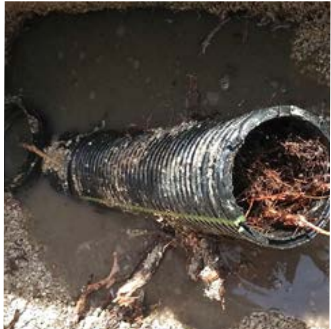
Clogged bunker drains cause serious issues. Companies can find and clear drains for you, or you can locate the clog and address the issue yourself.
