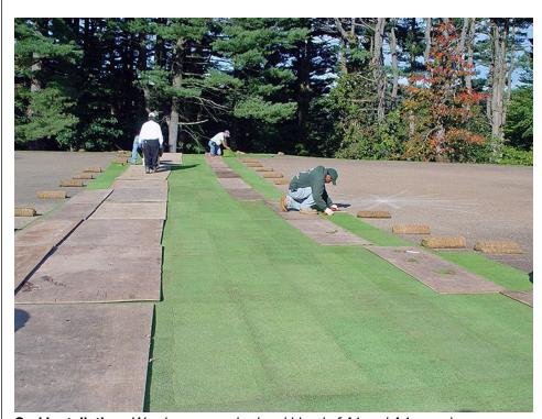
**Sod Installation:** We chose a washed sod blend of A1 and A4 creeping bentgrass from a commercial nursery in New Jersey. The grassing crew managed to install 10,000 square feet of sod in about six hours, working off plywood. We incorporated a granular organic fertilizer into the upper rootzone prior to the installation. The last green was completed on November 2, 2010.
