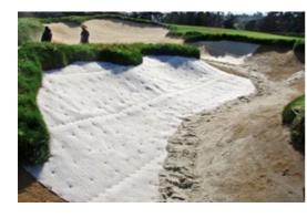
Bunker construction has become an increasingly elaborate and expensive process. The wide variety of bunker liners that are now used, and their rising costs, are indicative of this trend. Liners are intended to improve playability, reduce maintenance and extend the life of bunkers — all worthwhile objectives. Unfortunately, deciding which liner to use, or whether a liner is necessary at all, is not always straightforward.
