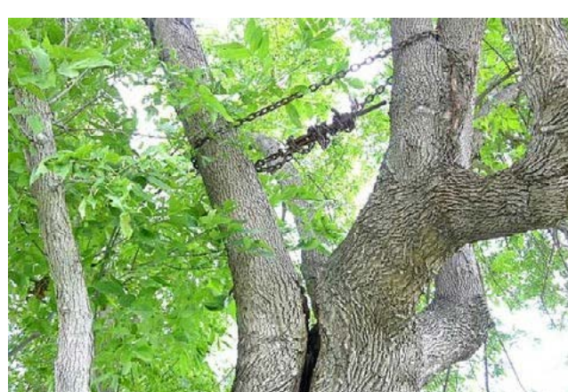
A comprehensive tree survey can provide valuable information on the proper way to brace and cable key trees as they age and which trees are good candidates for preventative maintenance procedures.
