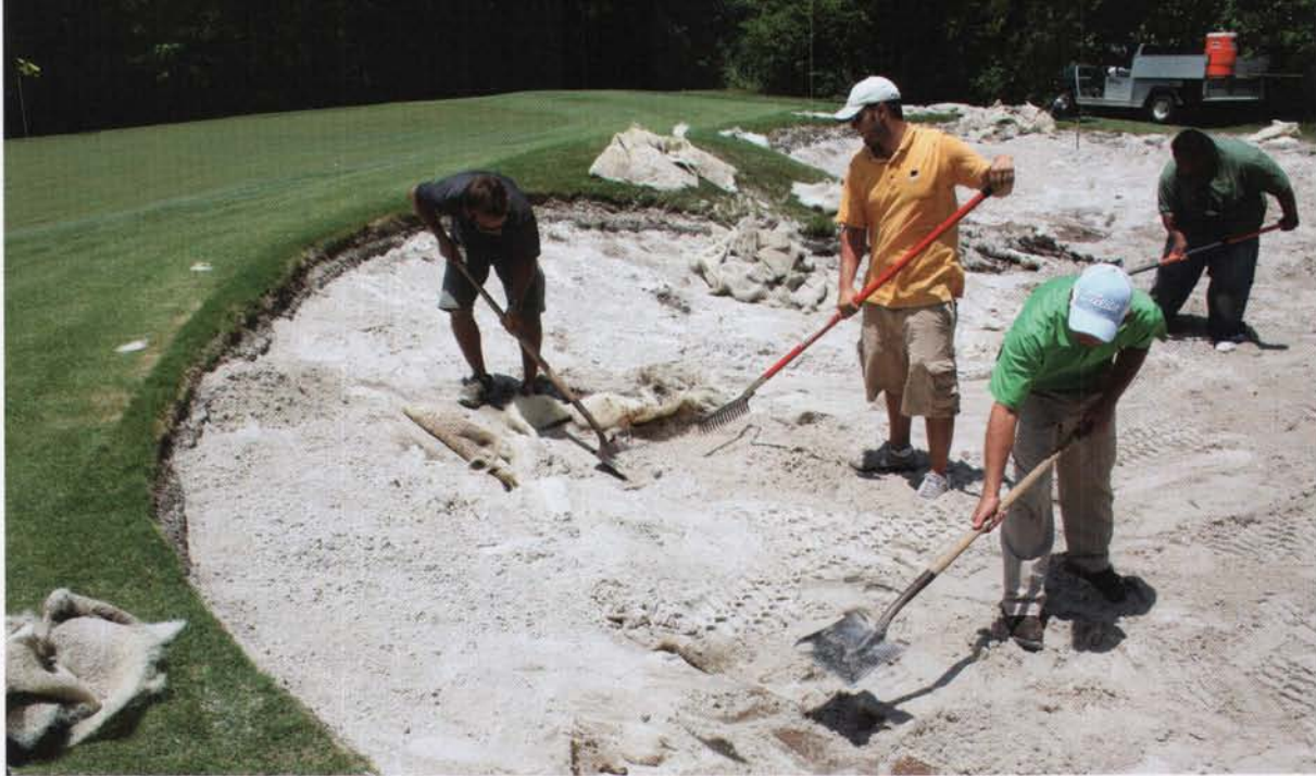
Bunker liners are not a cure-all. Unless a great deal of labor is expended to keep plenty of sand on the bunker face, the liner can become exposed and snagged by golfers. To prevent maintenance equipment from damaging the liner, labor-intensive hand-raking of bunkers is recommended when liners are used.
