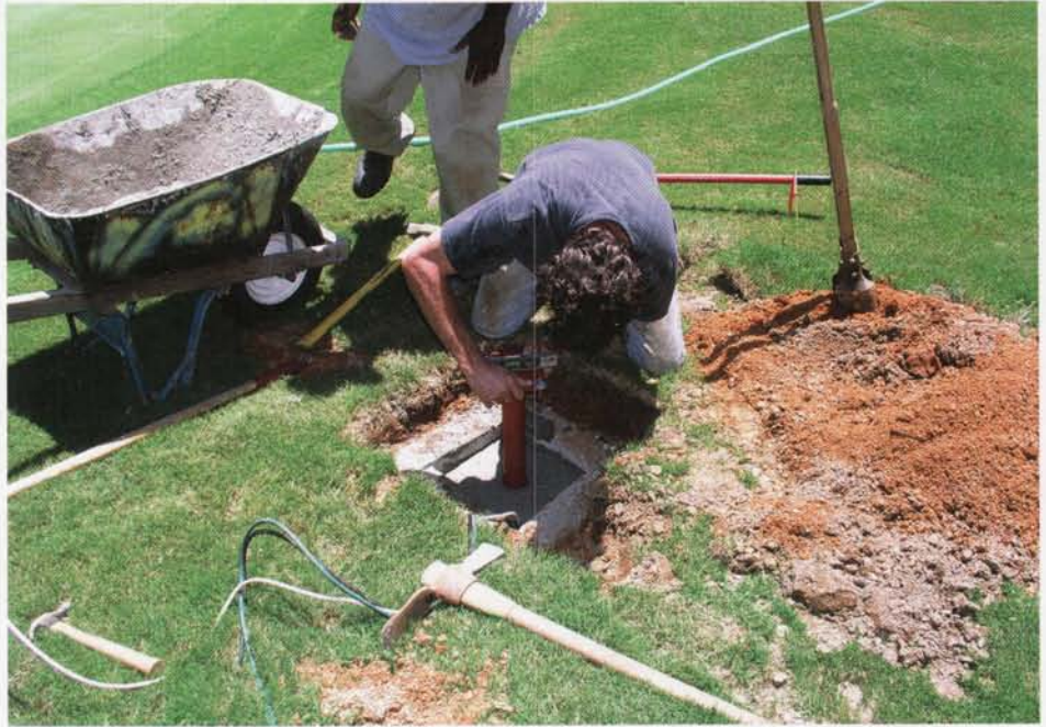
Above left: A combination motor starter and disconnect switch is installed on the upper fan pole on this three-phase motor fan. Since three-phase motors don't have thermal protection, it is essential to install these devices to protect the fan motor. Above right: Concrete is used to secure the four-foot ground pole that attaches to the fan pole. The concrete provides a long-term stable foundation for the fan.
