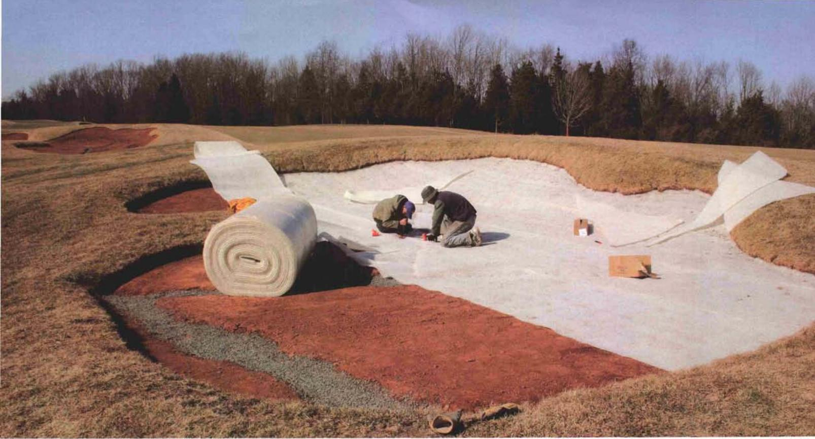
to keep enough sand over the liner to prevent players from contacting it during a shot. The goal is to maintain a depth of 1 to 2 inches on the bunker faces. To achieve this goal, the depth must be checked weekly and reestablished with hand shoveling as necessary.
