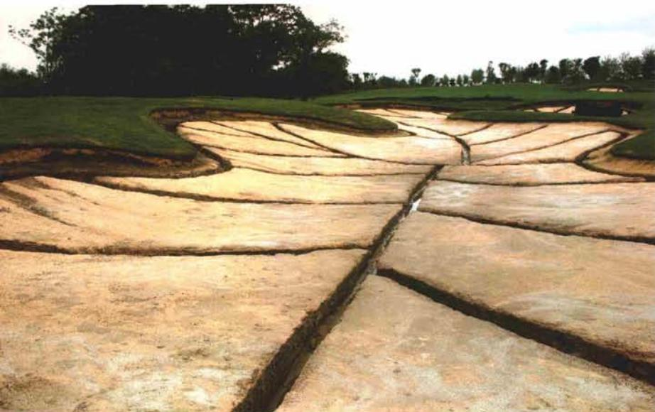
Drainage is critical in every bunker construction project and typically costs approximately \$5.00 to \$6.00 per linear foot.
