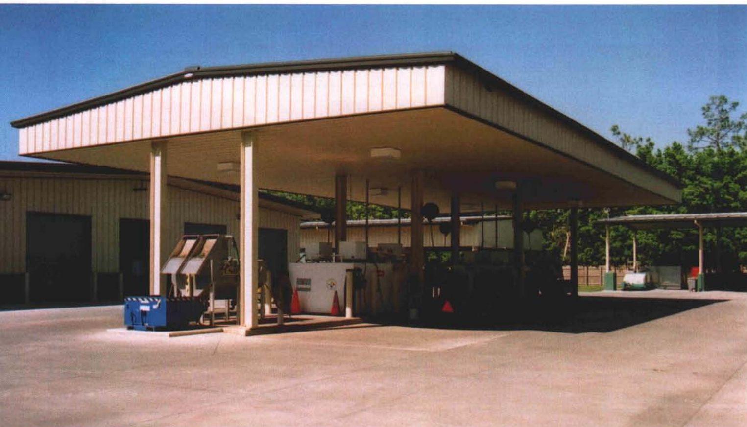
The golf course maintenance facility itself is an important component in the overall environmental management system.
