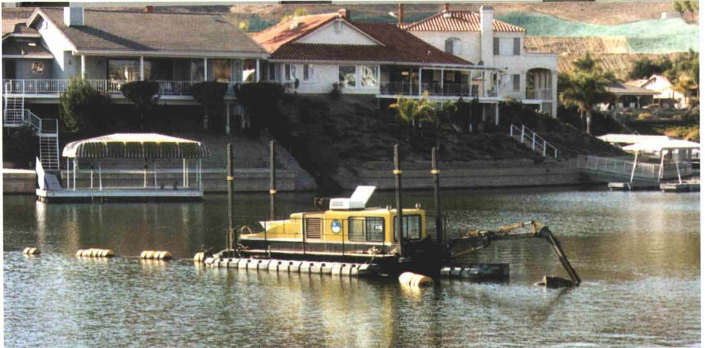
The hydraulically powered suction-head dredge vacuums sediment from the bottom of the lake and pumps the slurry to the processing area one-half mile away.
