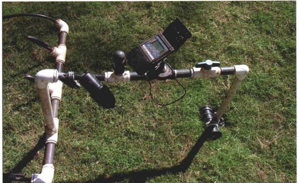
The Turtle Bay Golf misting system is adapted to larger sites with multiple lines sent from the control system. The lines have been pressure reduced from the regular irrigation system.
