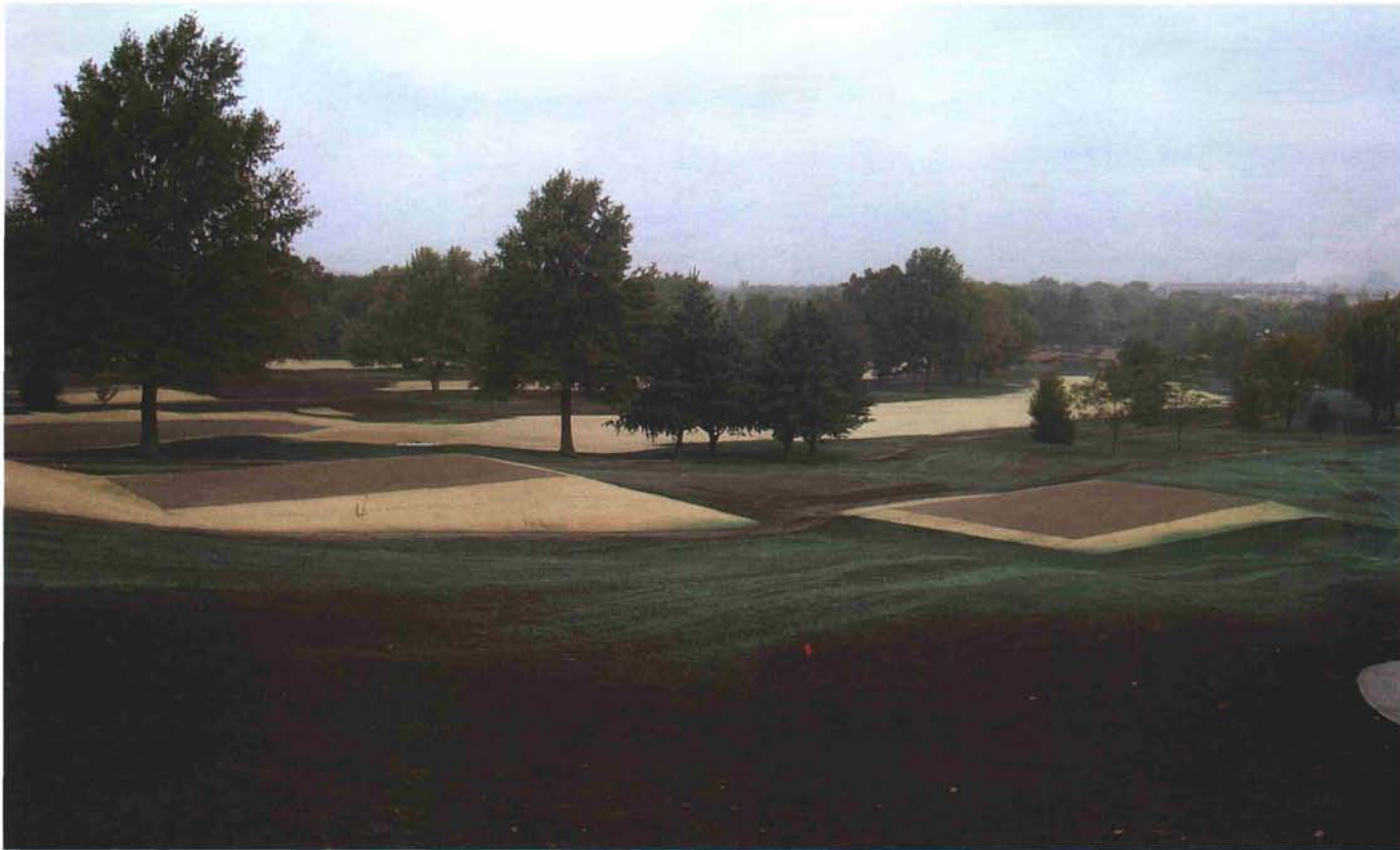
With improvements in erosion control blankets, their use on new construction sites is on the rise. In addition to being less expensive, high-quality blankets extend the establishment window of cool-season turf species and provide better-than-expected ground stabilization.
