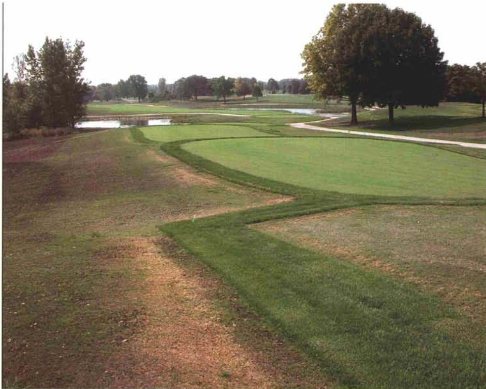
One of the most common methods for controlling soil erosion and establishing a stable worksite for equipment operation is to surround newly constructed areas with sod. Given recent improvements in erosion control blanket technology, however, superintendents can do equally well with seeding.
