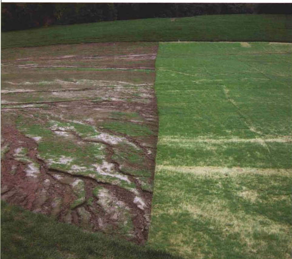
Taming soil erosion on new construction sites, superintendents, architects, and golf course builders are turning to the use of improved erosion control blankets.
