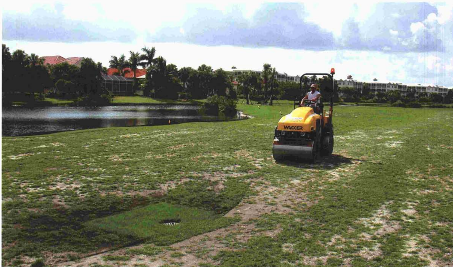
Playing surfaces were rolled multiple times to provide smooth, uniform playing conditions.
