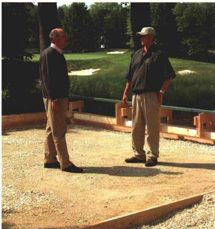
An occasional tour of the course allows the green chairman to learn more about on-course activities. In this case, two sand storage platforms are being built in key locations to facilitate easy replenishment of sand for topdressing fairways.
