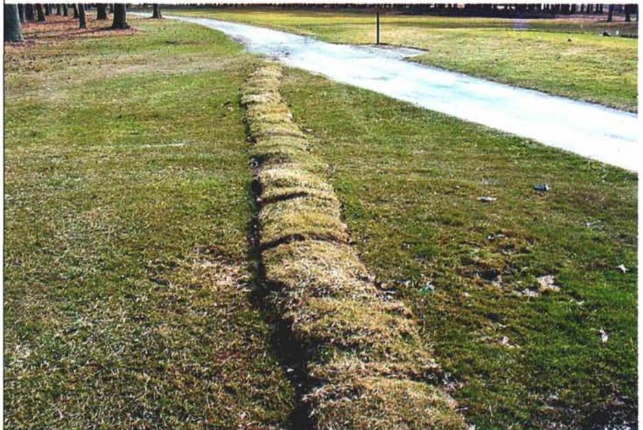
Just mounding the trenches and waiting for settling is not the proper installation technique. New and existing grades should be evenly matched.
