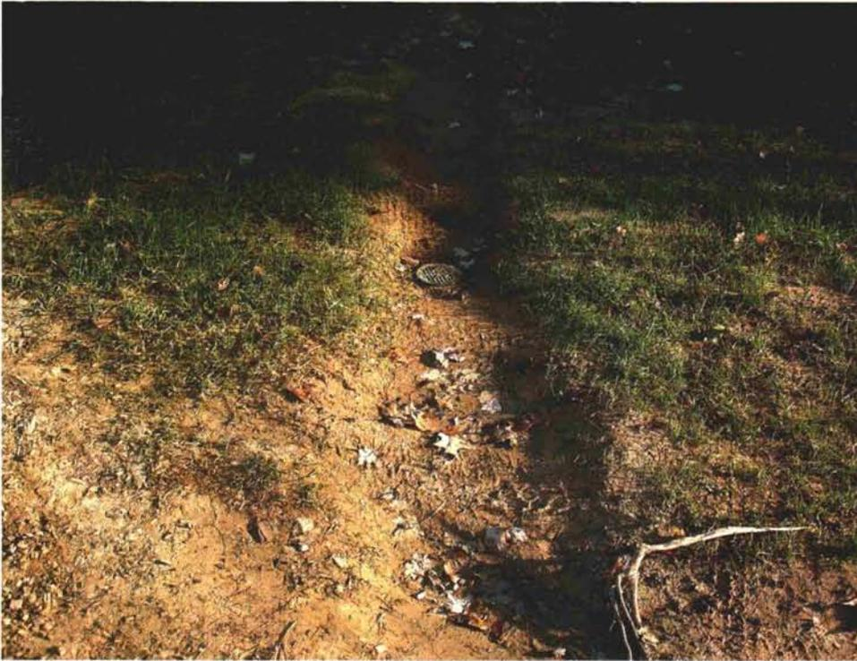
Trench settling will be obvious for years, and therefore trenches need to be properly compacted during installation.
