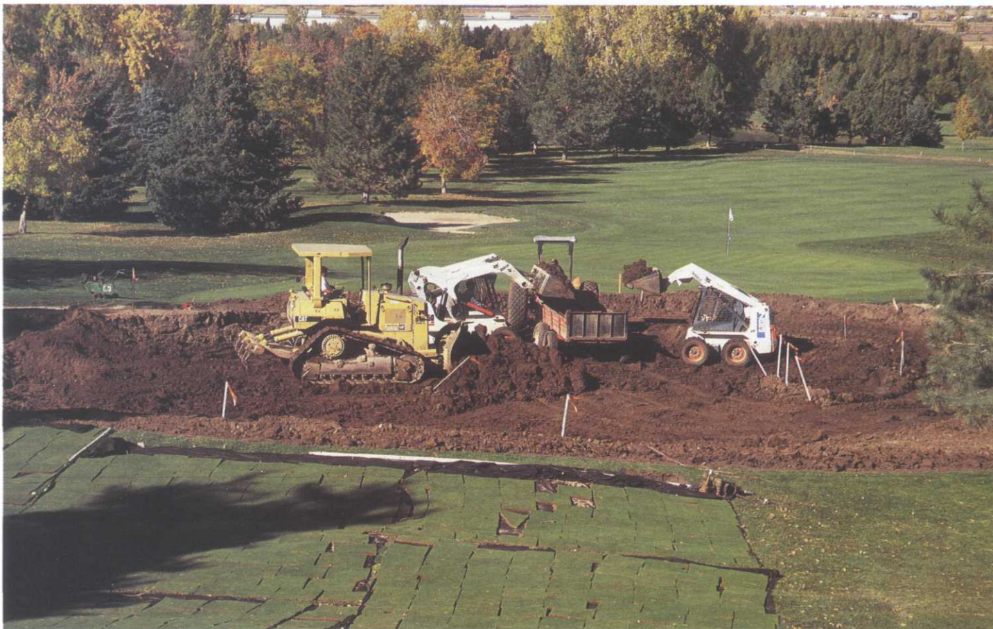
Putting green reconstruction involved minimizing disturbance to the surrounding area. Notice the putting green turf that has been stripped and set aside on plastic for reuse.
