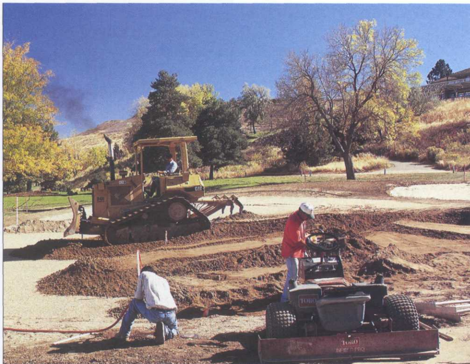
The new greens were designed to preserve design integrity and character while softening slopes to increase the number of hole locations. They were built to USGA Guidelines for Putting Green Construction.
