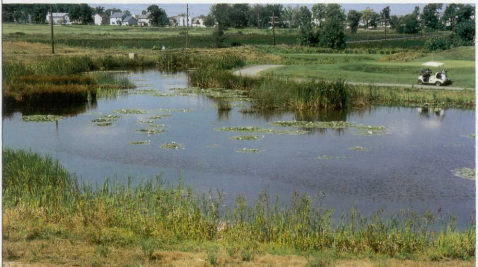
Unlike stormwater retention basins, a wetland cell with active plants and anaerobic sediments will have a significant retention and degradation capacity for introduced materials. The created wetland system in the Purdue University research study was efficient at improving water quality.
