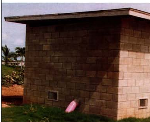
It is commonplace that purple irrigation system components generally signify and warn unsuspecting users of the presence of recycled water.
