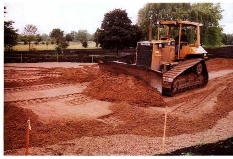
The gravel layer continues to be an integral drainage component of USGA greens. Scientific research has demonstrated another important function of this layer — to help equalize moisture retention levels throughout the green.
