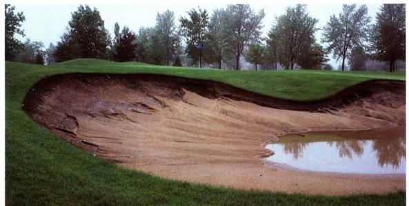
Left: Poor construction or design can lead to serious drainage problems after wet weather and results in more of a penalty than necessary.
