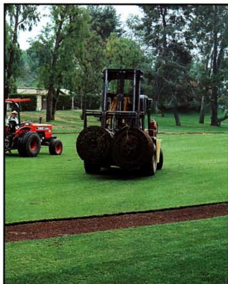
One method of renovating fairways is to strip out the common bermudagrass and then install big rolls of hybrid sod. Half of a fairway can be converted at a time to allow play to continue. See page 13.
