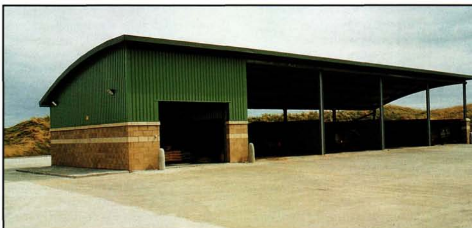
An open storage area can be used to house materials and equipment that needs to be covered but not completely enclosed.
