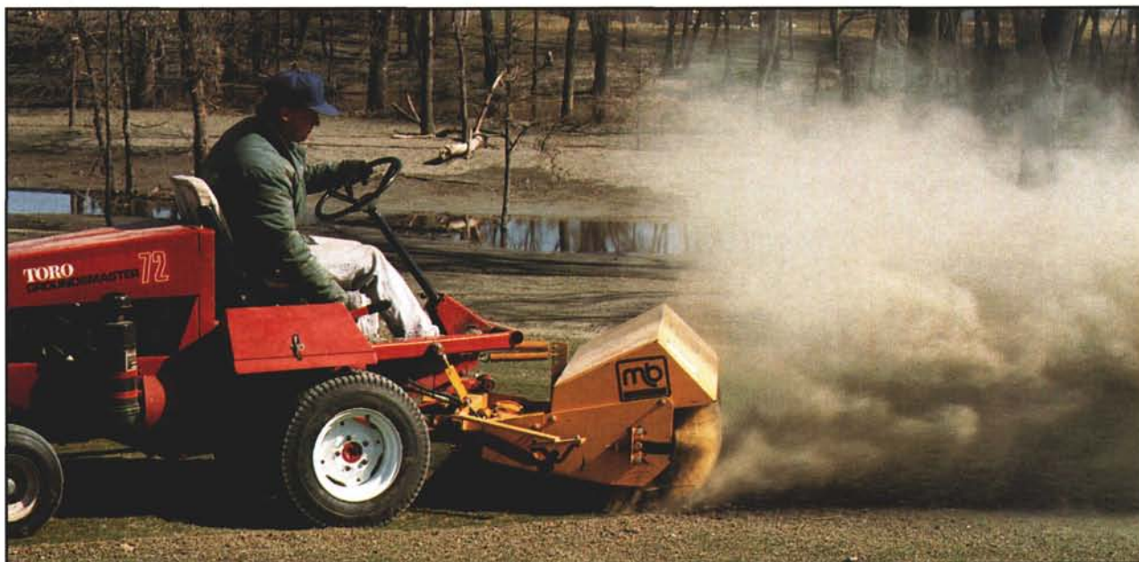
In places where silt deposits were thin enough, mechanical brushing was sufficient for removal.
