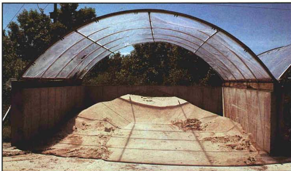
A plastic-covered roof can readily be installed over existing topdressing bins to provide effective protection from the elements.
