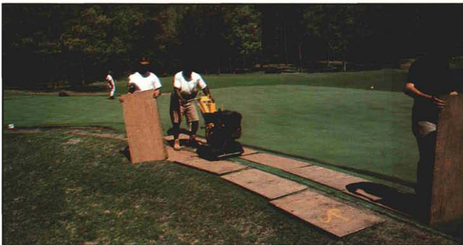
The Greens Encroachment Barrier System is installed in 100-foot sections using a vibratory plow.
