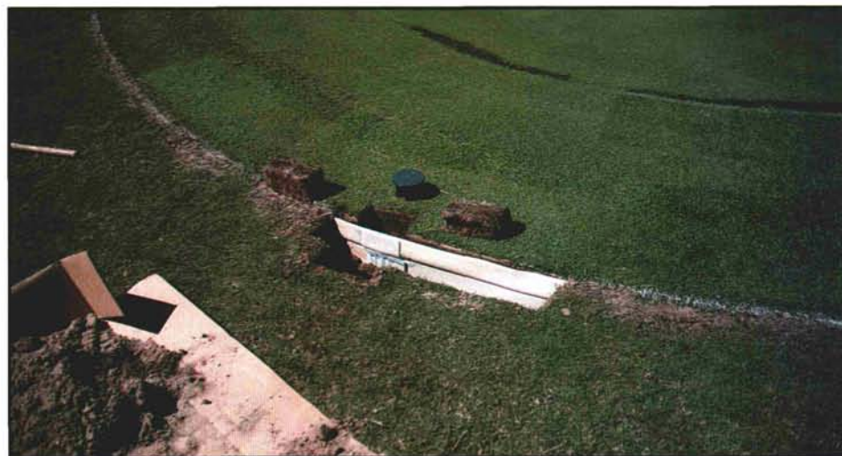
The 8-inch depth of the barrier blocks rhizome movement into the green and can act as a wicking barrier between green rootzone material and the soil in the surrounds.
