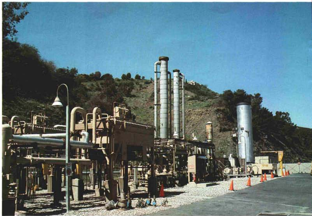
(Above) Methane, a large component of landfill gas, can be captured and used as a valuable energy source. This processing plant at Mountaingate Country Club in Los Angeles processes methane for use at the nearby UCLA campus.
