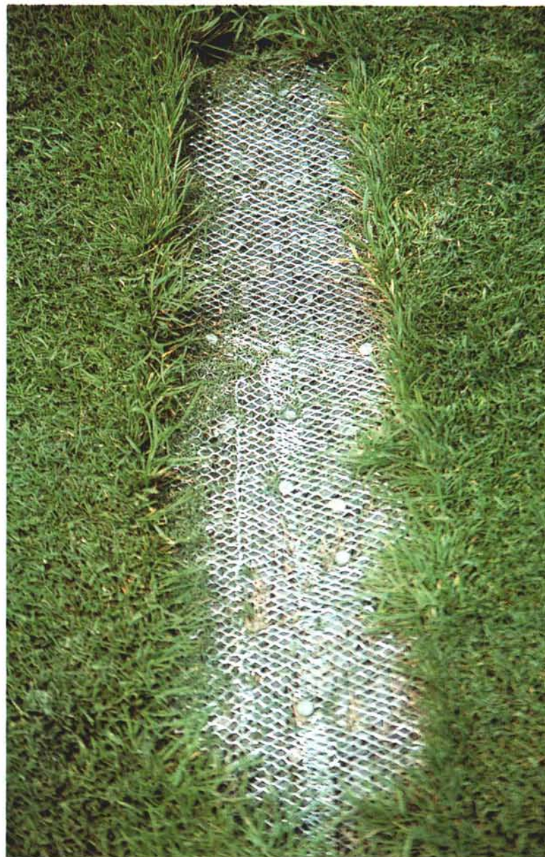
Gutter Guard holds stones in place and encourages the grass to grow over more quickly.
