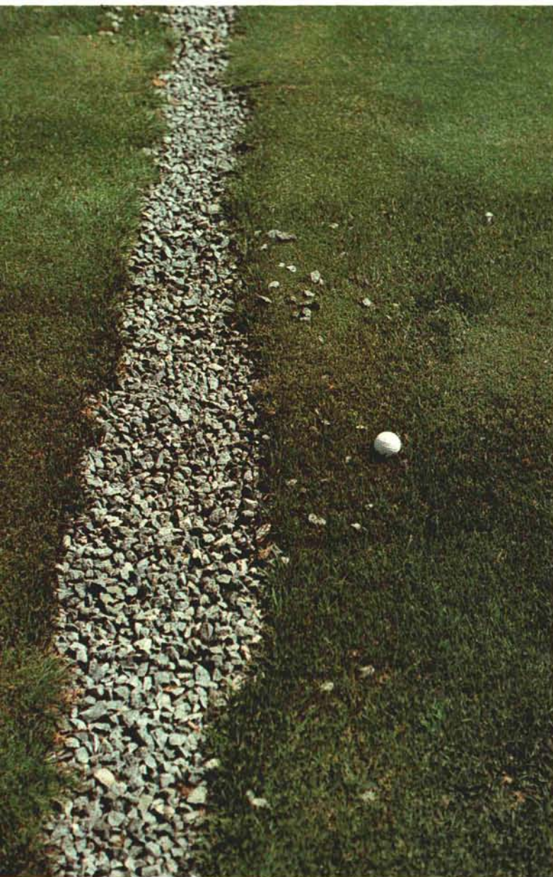
Open stone drains are effective, but dislodged stones are a nuisance.
