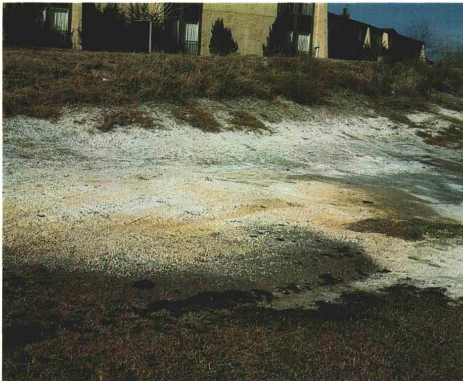
Calcium and magnesium salts accumulated along a seepage zone next to the cart path. Seepage occurred from excess irrigation applied to the adjacent landscaping.
