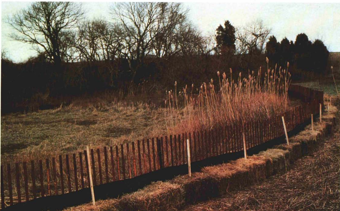
Erosion control methods employed around the wetlands.
