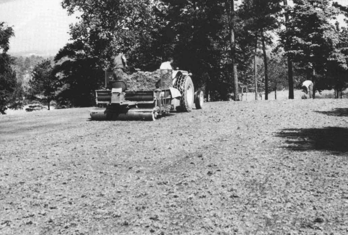
Greens were replanted rapidly where large equipment was utilized.
