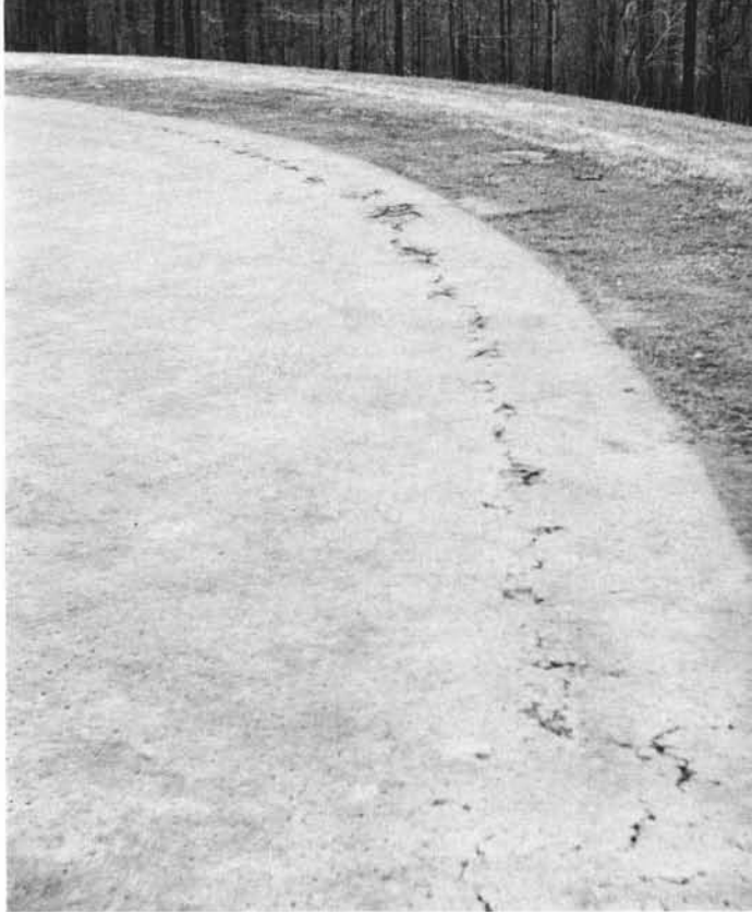
Greens dry from the edges first because of soil texture difference between the green proper and the collar. Drying occurs in winter as well as summer. Severe desiccation caused cracks in edge of the green above.
