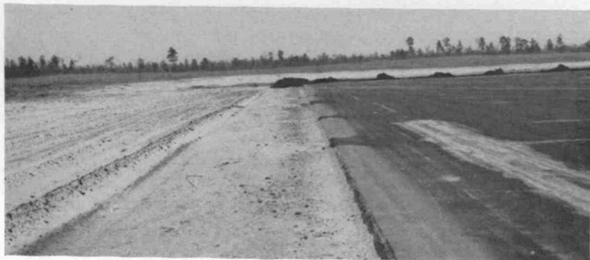
Trench 10 feet wide at the edge of an airfield runway excavated in preparation for "mucking." A 4 to 6-inch layer of muck is used to fill the trench. Natural vegetation growing in the muck is expected to produce a dense cover along the edge of the runway. The muck has already been placed in the trench in the background.
