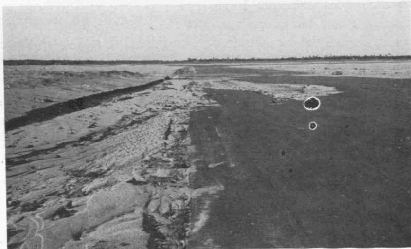
Result of lack of grass cover on airfield. Note the soil which has been washed onto the runway from adjacent bare areas. Such a condition might be prevented if a good grass cover were established.
