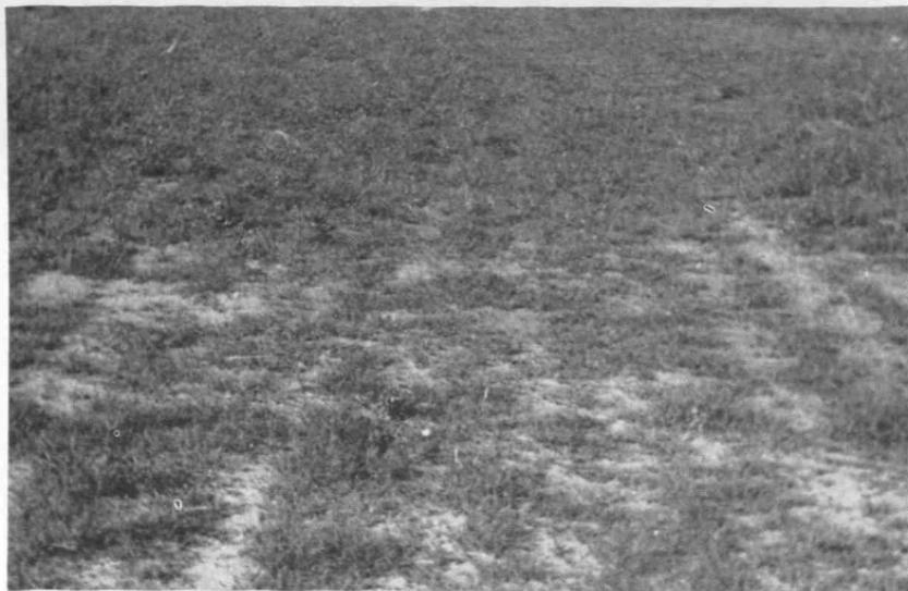
Bermuda grass turf which has been sprigged on an airfield. Foreground, on subsoil; background, on topsoil. The difference in amount of vegetation in the two areas is due to a larger number of annual weeds on the topsoil in the background rather than to a heavier stand of grass. Weeds retard the growth of grass and then die in late summer or early fall. A poor cover will remain on the area in the background after the weeds have died.
