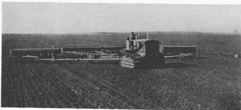
Large scale seeding and fertilizing may be accomplished in one operation by the use of tractor-drawn drills.
