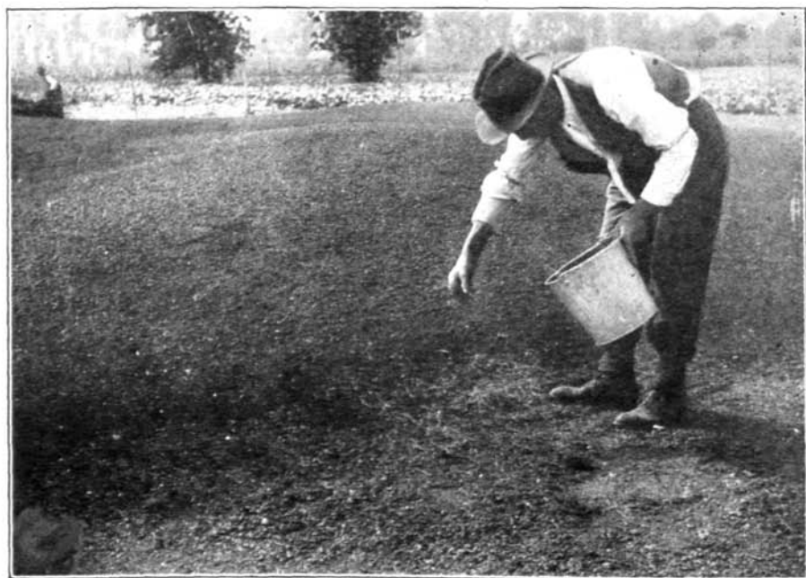
Scattering the pieces of stolons for sod. The top-dressing has been spread in the background, but not rolled.
