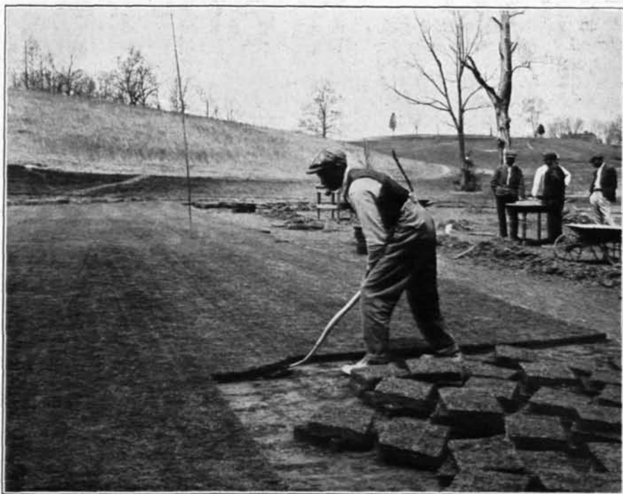
Fig. 2—Lifting Sodds With Hand Tools
