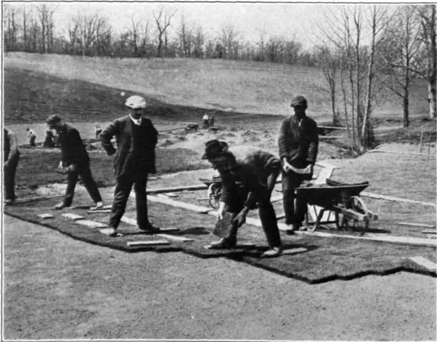
Fig. 3—Laying the Sods on a Green Courtesy of Macmillan Co.
