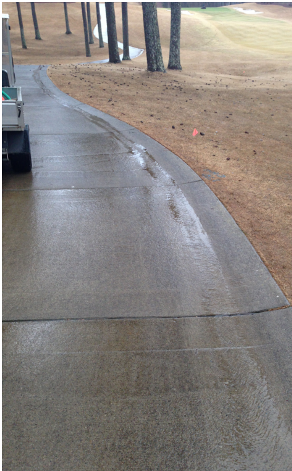
Curbing along a cart path can collect surface water and divert it away from playing areas.
