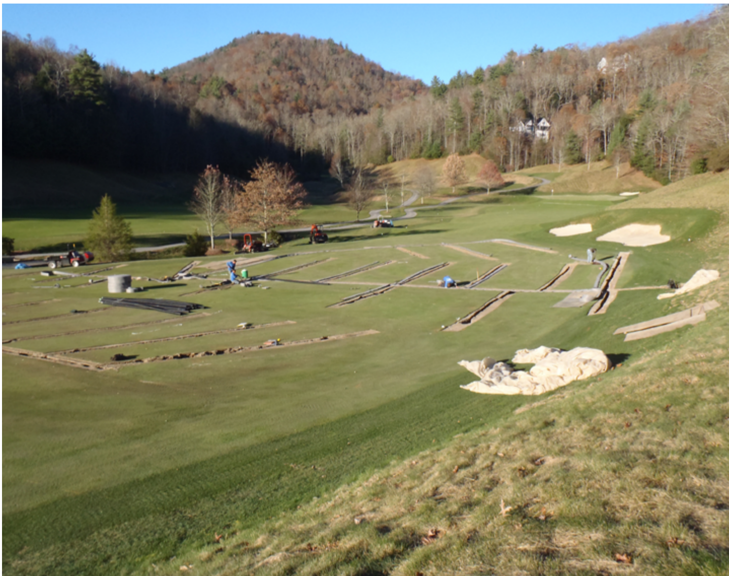
Extensive drainage improvements may need to be done in phases, so proper planning is essential.
