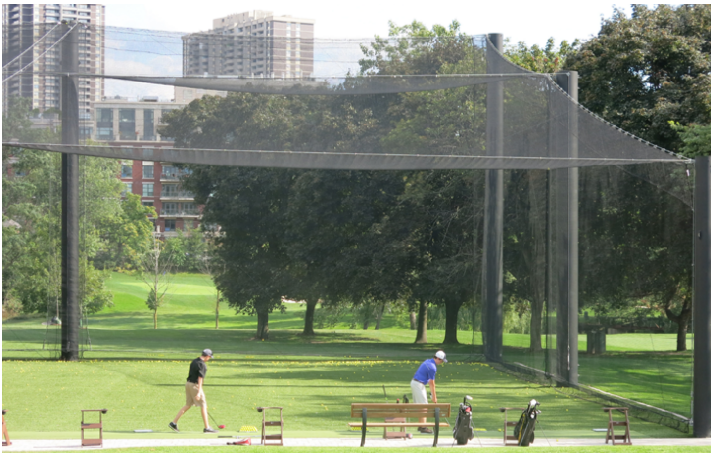
Netted facilities can provide an excellent practice experience at golf courses where there is not enough room for a full-sized driving range. When the ceiling net is angled upward, golfers can watch the trajectory of their ball flight.
