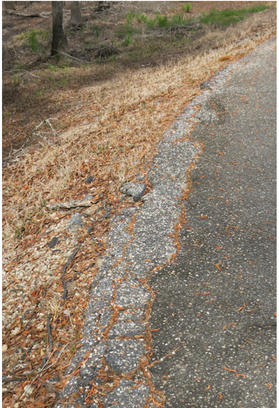
Traffic from golf carts and maintenance equipment can quickly break down cart path edges when paths are not sufficiently wide.
