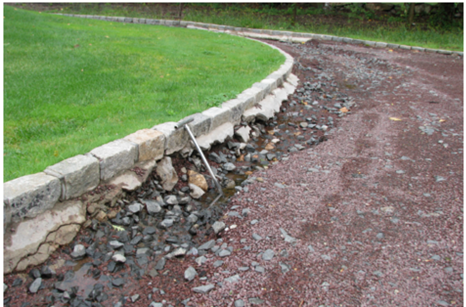
Cart paths constructed from unstable material may wash out and require significant time and money to repair.
