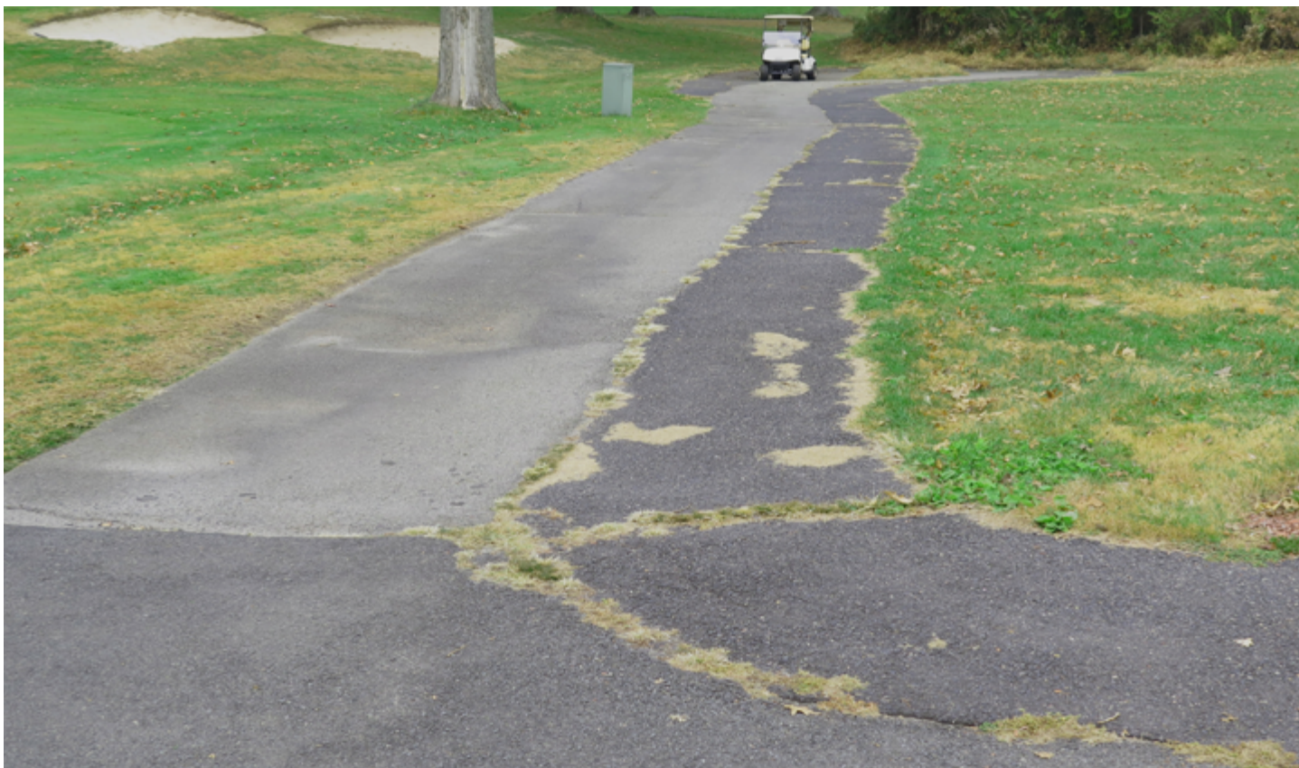
Paths that are too narrow initially must be widened to accommodate traffic.
