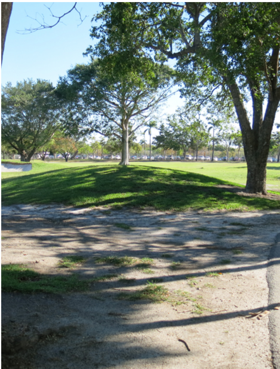
Concentrated traffic entering or exiting a path leads to predictable turf damage. The presence of trees in these areas makes it almost impossible to maintain turf cover.
