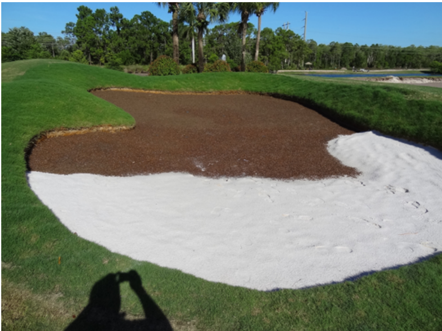
Sand being installed atop the stabilized gravel liner of this Better Billy Bunker™.
