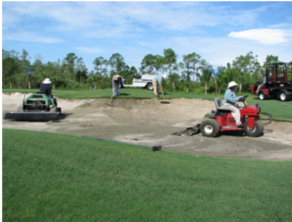
Flashed bunker faces provide a certain architectural appeal, but they require more maintenance to relocate sand that washes downward following rainfall.
