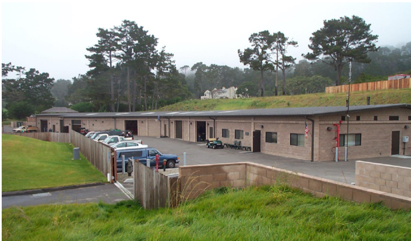
A clean, organized, and well-designed maintenance facility will bolster employee morale and efficiency.
