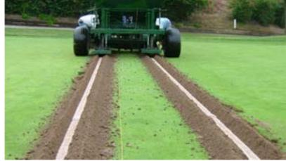
Installing sand-channel drainage can improve the performance of poorly-drained areas, but special attention must be paid to the physical properties of the backfill material to ensure best results.
