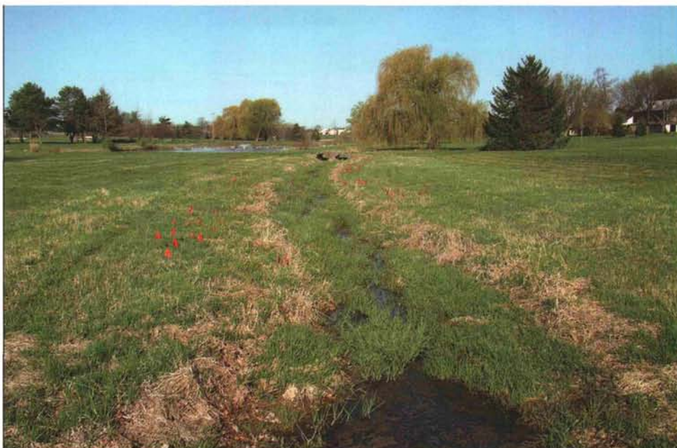
With just a few phone calls and some coordination meetings, Elks Club now saves about $5,000 per year in reduced maintenance costs.
