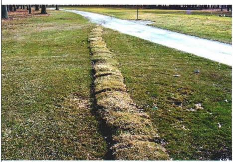
Just mounding the trenches and waiting for settling is not the proper installation technique. New and existing grades should be evenly matched.
