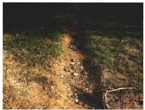
Trench settling will be obvious for years, and therefore trenches need to be properly compacted during installation.
