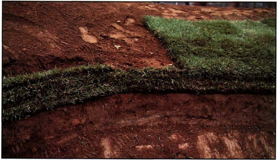
The final step was to position a full piece of sod perpendicular to the stacked sod along the edge of the bunker. The perpendicular sod pieces provided a cap for the stacked sod.
