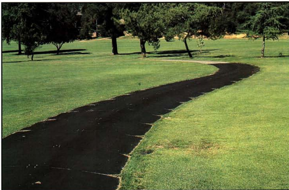
There is no perfect cart path surface for all situations, but rubber horse stall liners have provided a durable, low-bounce cart path surface at Cameron Park C.C. (Cameron Park, California). Road base was installed on the subgrade of the cart path with a railroad tie embedded along the midpoint. The railroad tie was used as a contact point for the rubber mats and to provide a crown to the surface.
